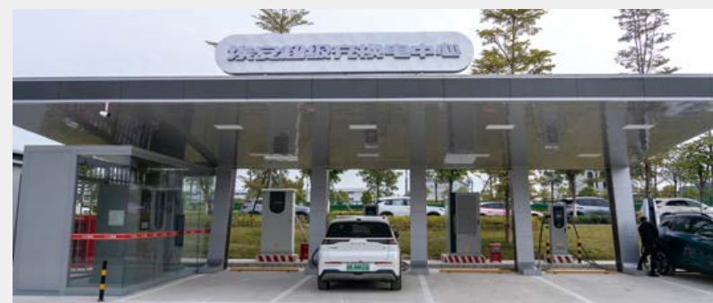
Charging and Switching Center
