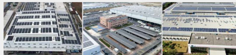
Construction of Photovoltaic Projects in Parks of GAC Component
